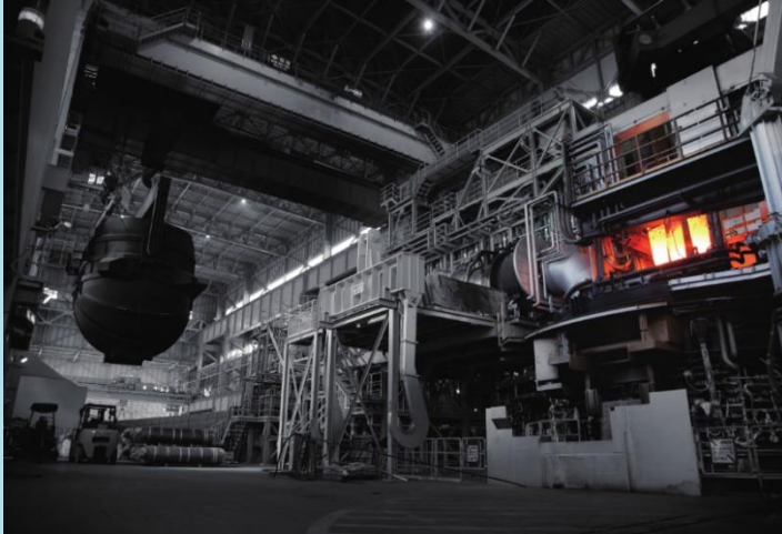
Electric arc furnace with rotating drives, operating at our Chita Plant (STARQ®)
