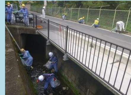
Shibukawa Plant: Community cleanup
