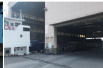
All-weather berth loading
