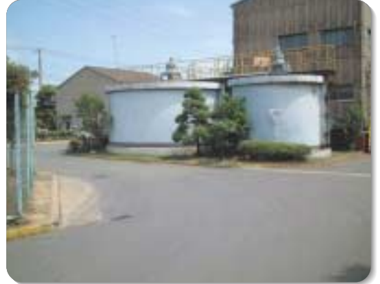
Drainage processing equipment (Kawasaki Plant)
