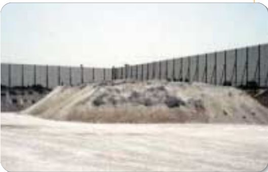
Fence around slag dumping/recycling treatment yard
