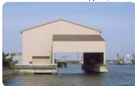
All-weather shipyard (Chita Plant)
