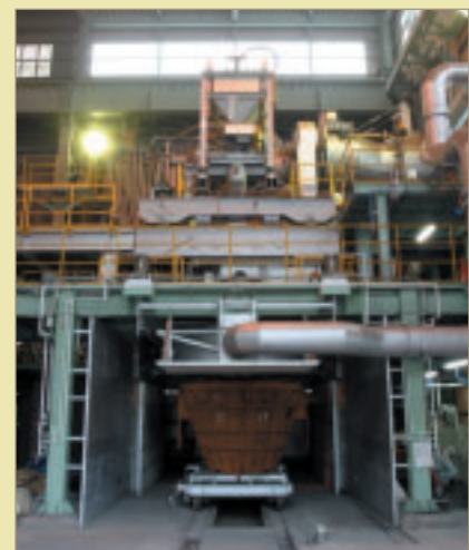
A DSR furnace
