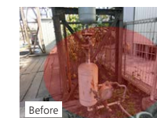
Possible to confirm air leak, but precise location unclear
